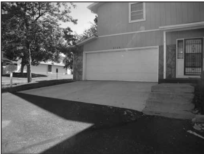
New asphalt at 2724 South Xanadu Way.
